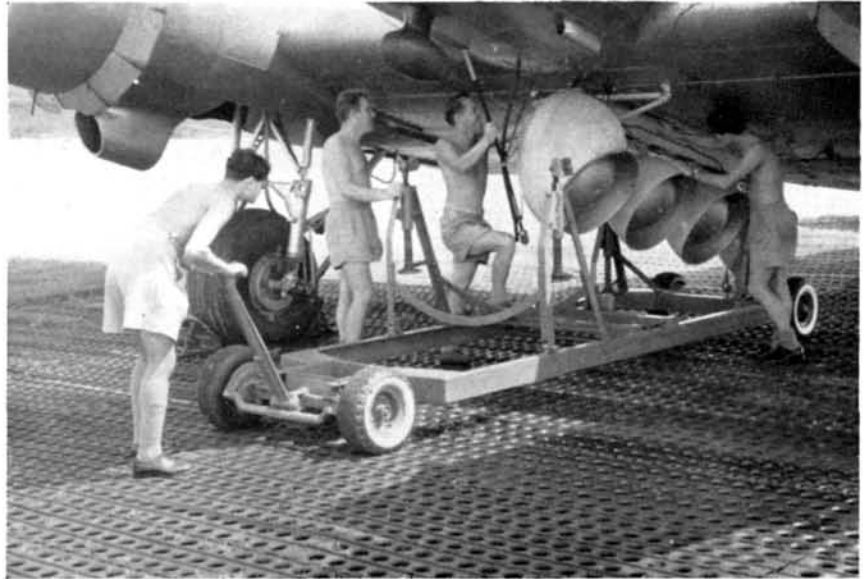
Here the boom trolley is being removed from the Dakota. Left to right are: L.A.C. Ghodgoanikar, Sgt. G. J. Winsley, SAC. R. D. McMurrie and JT. P. Pyke.
